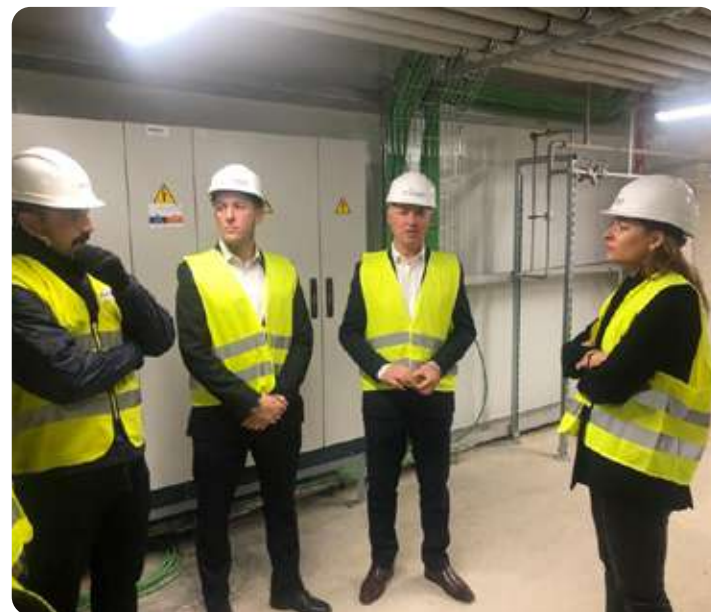
Esther Muñoz visited the works at Vivunt Pharma in Villadangos del Paramo.
