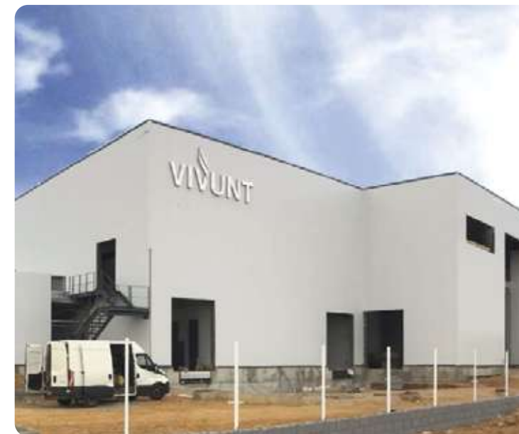
Works at the factory in Villadangos del Paramo (Leon).
